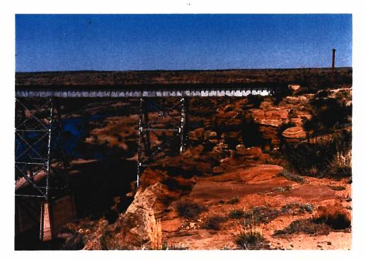
Photograph 13 – Lake Meredith Salinity Study – Logan, New Mexico Area – View looking east (downstream) along the Canadian River trench. South abutment of railroad bridge shown anchored to Trujillo Sandstone (SW 1/4 sec. 14, T. 13 N., R. 33 E.).
